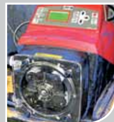
LPP-M pumping sodium hypochlorite 12.5% at Nashua New Hampshire.
